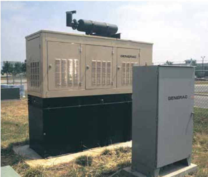
The runway lights, instrument landing system and navigational equipment are backup up by this 100 kW unit.
