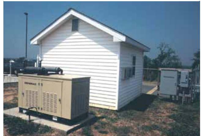
The runway lights, instrument landing system and navigational equipment are backup up by this 100 kW unit.
